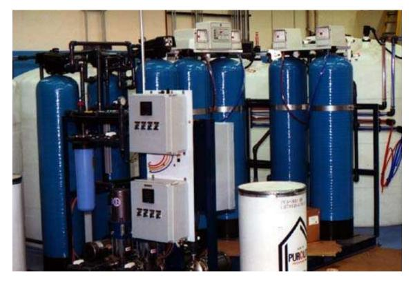
Ion Exchange Units Ion exchange technology is one method to remove Arsenic from drinking water
