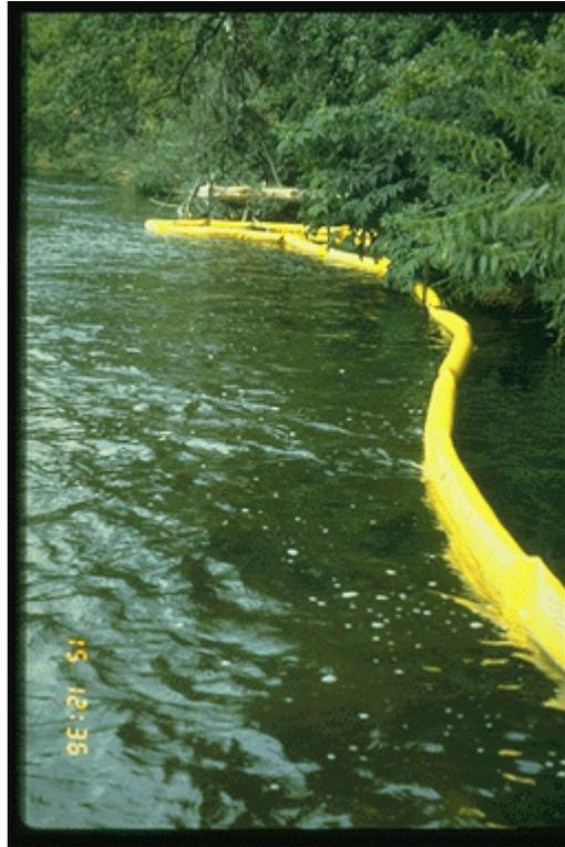
An absorbent boom on a surface water body to prevent migration of oil.
