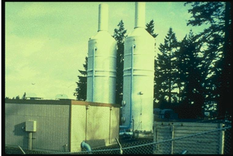
Twin air-stripping towers for treating contaminated groundwater.
