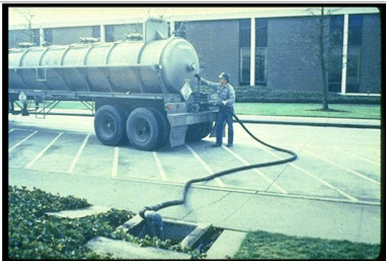
Vacuum truck extracting fluids from a monitoring well.
