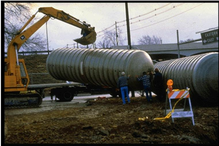
Fiberglass-reinforced plastic (FRP) tanks being offloaded from a transport truck.
