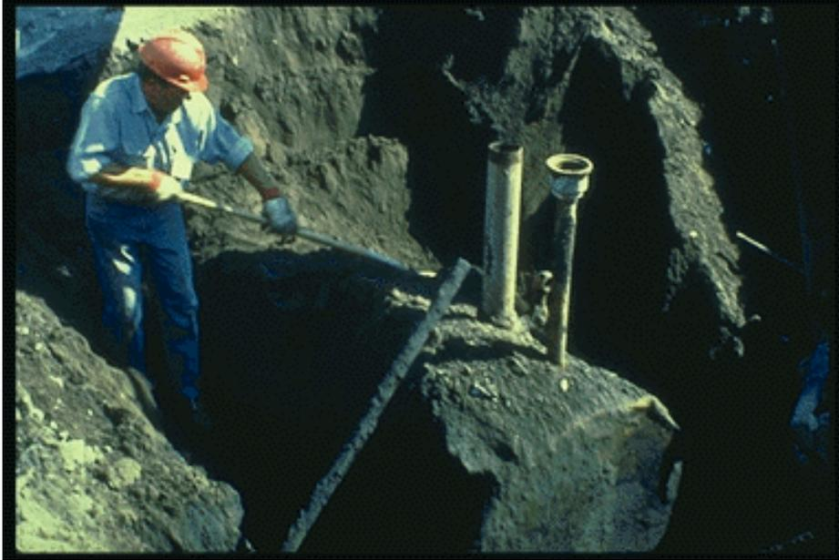
Manual labor during an UST excavation. Beware of toxic gases and install shoring where needed.
