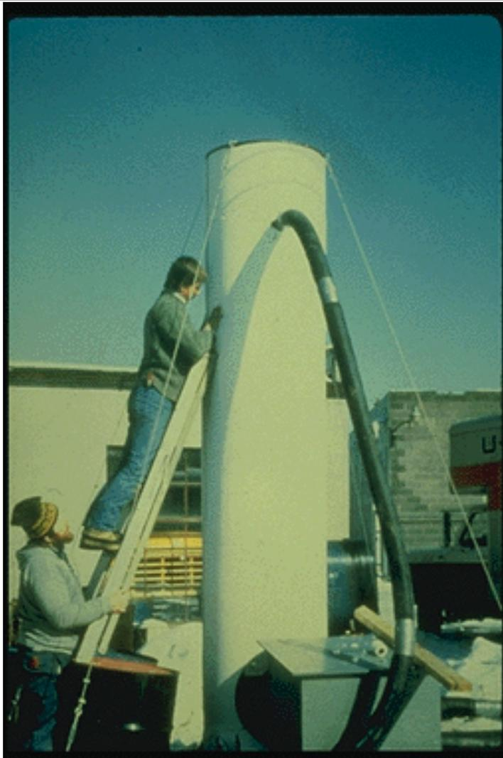
Air-stripping tower for treatment of contaminated groundwater.
