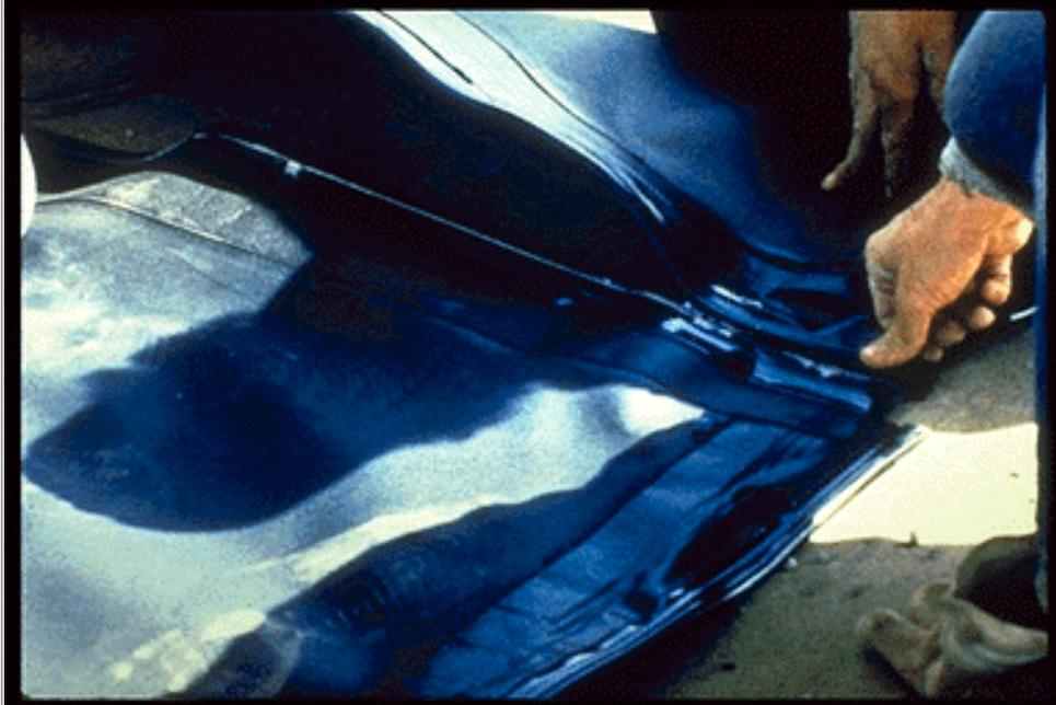
Bonding the seams of an excavation liner.
