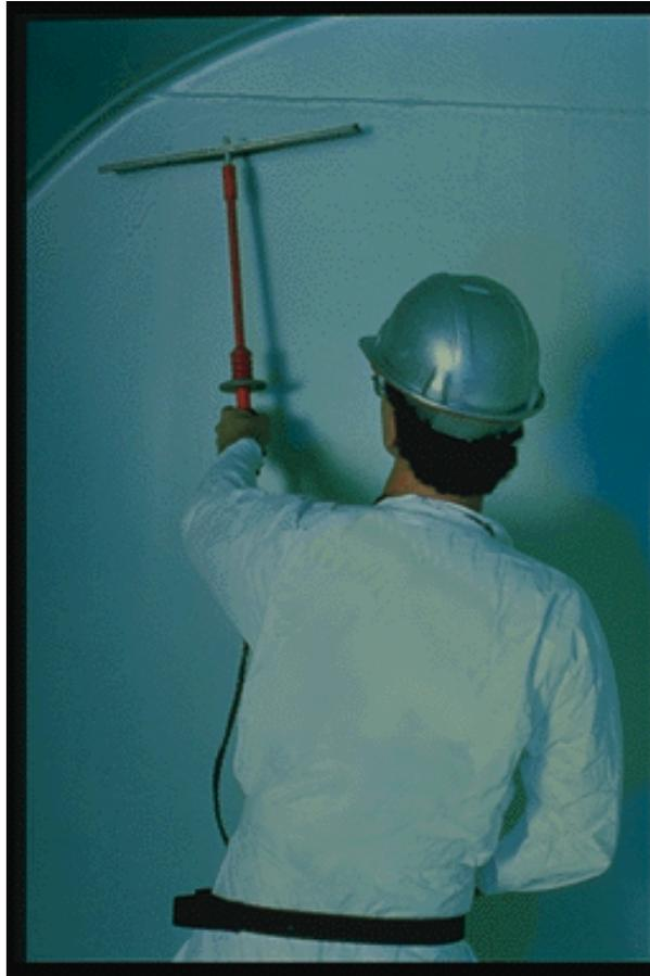
Checking for "**holidays**" in a recently applied tank lining.
