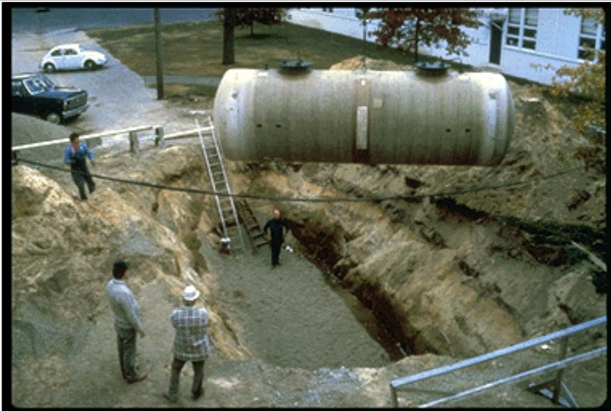
Lowering a fiberglass tank into an excavation.
