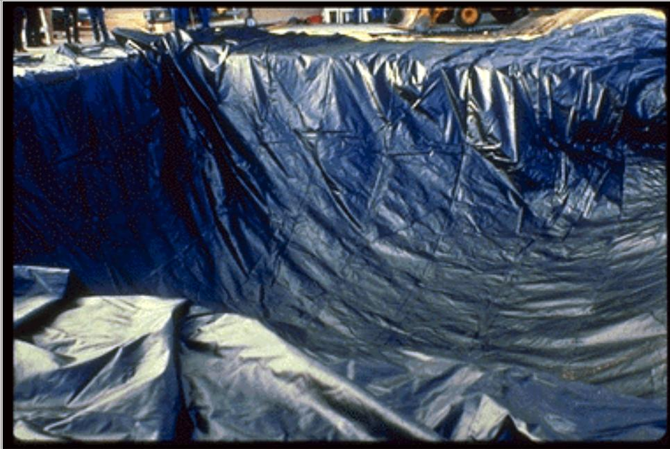
An impermeable excavation liner.
