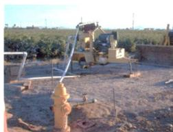
Direct connection from hydrant to pump.
