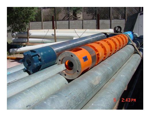
A new 8-inch submersible pump and motor with 6 inch column pipe about to be installed in a high capacity municipal supply well.
