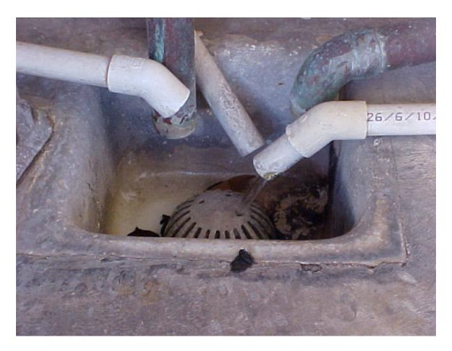
Which of these ice machine drains has an approved air gap? Here is a better question; would you use the ice from this ice machine? Here is where all those stories about cockroaches and stomach flu originate. The stories are true.
