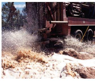
Jetting Nozzle that can be → attached to drill pipe.
