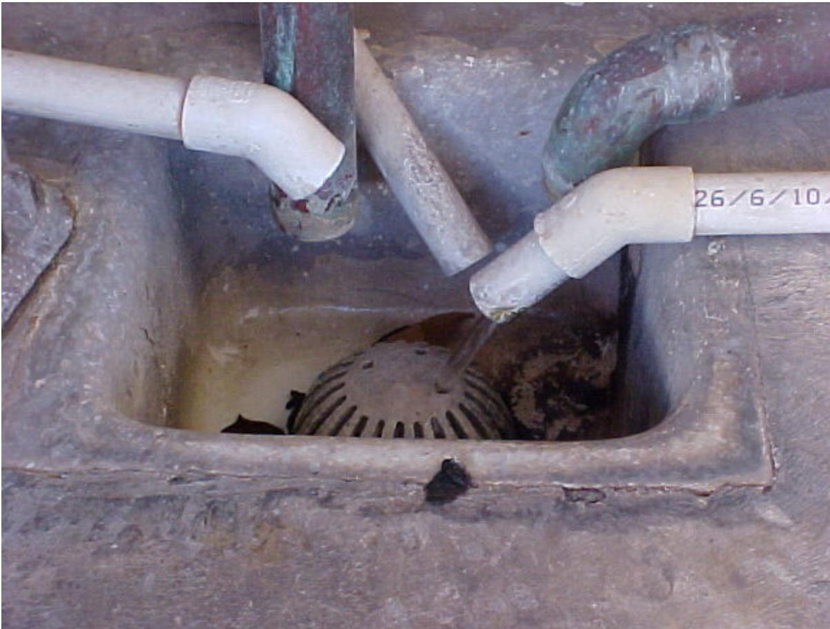
Which of these ice machine drains has an approved air gap? Here is a better question; would you use the ice from this ice machine? Here is where all those stories about cockroaches and stomach flu originate. The stories are true.
