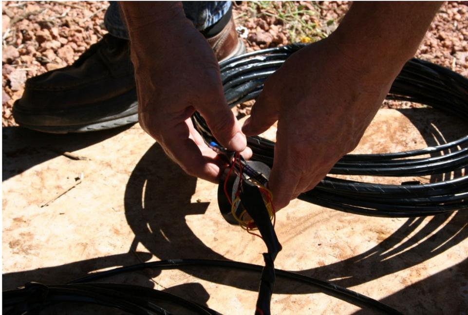
Preparing an explosive charge to 'hydrofract" or loosen or dislodge any debris or corrosion inside an existing well casing. This explosive material is made in 25 or 50 foot lengths and has a blasting cap to start the explosion. Believe it or not, you cannot hear the explosion, since it is deep underwater. The bottom photo is the remains of the explosive charge. This procedure will usually increase well production.
