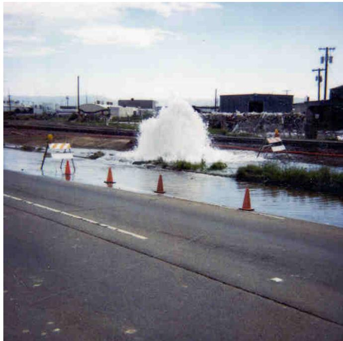
Broken water main, much larger and stronger leak, more damage, more customers without water. More chance of water contamination.
