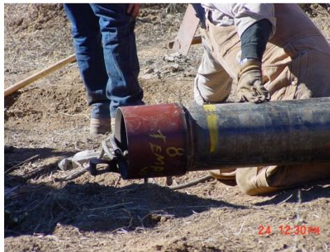
Cutting Shoe: The Cutting Shoe is welded to the bottom of casing before installation.
