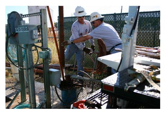
Top, this crew is removing a pump from a contaminated groundwater well in hopes of rebuilding and cleaning the well to increase the water production. The water is then sent to the granular activated carbon (GAC) vessels in the lower picture for final cleaning before being delivered to water customers. This well was contaminated from the dry cleaning chemical known as Perc (PCE) or fugitive Tetrachloroethylene from a nearby Dry Cleaner facility.
