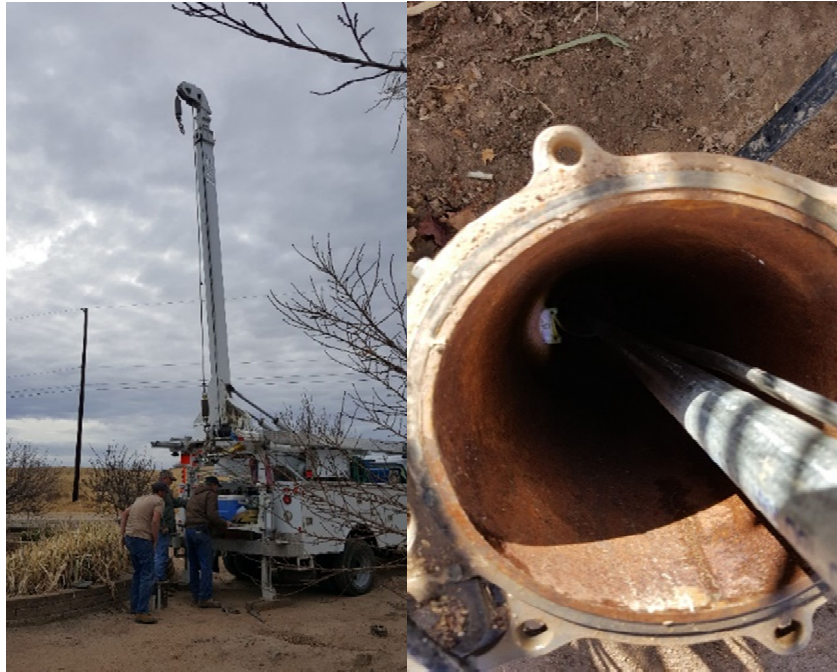
Well cap removed, looking at pvc pipe and electrical wire
