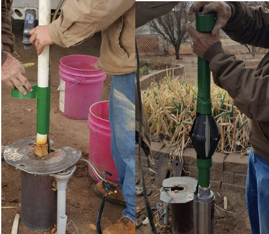
Installing new submersible pump, securing wire and connecting pump wiring.
