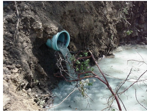
Last Pit (small amount of fines)
