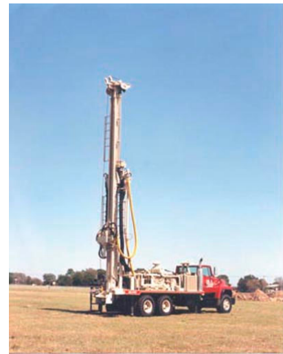
Typical Rotary Rig
