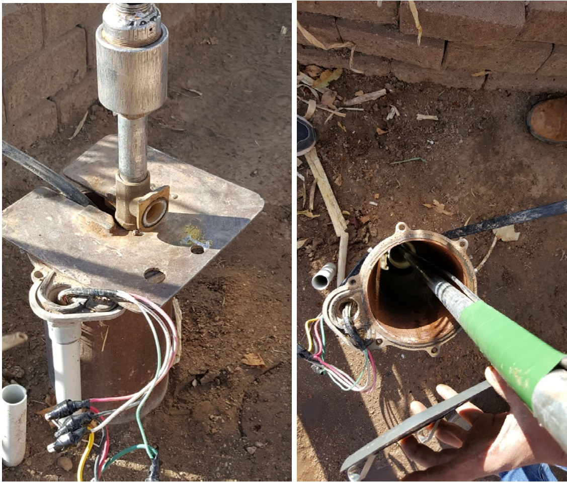
The discharge side of the pipe has a tee that seats on a saddle down below ground to prevent freezing.
