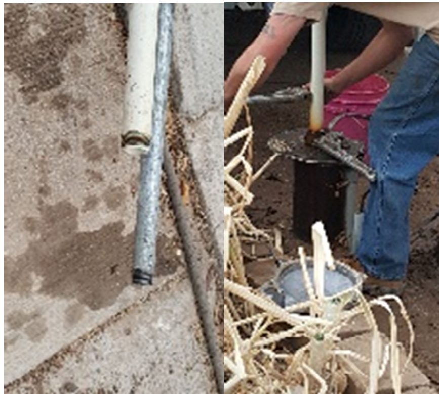
Attachment that screws into well pipe to be pulled. Metal disk supports couplings on wellhead while being pulled.
