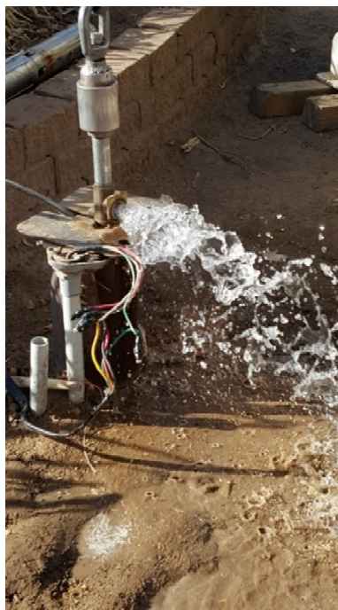
Checking to make sure new pump is working properly.
