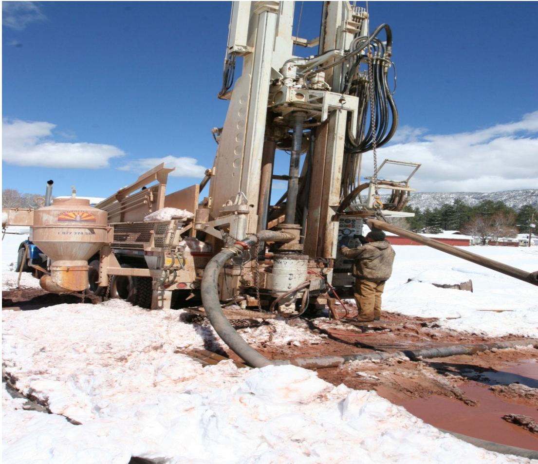
A drill rig in the snow.
