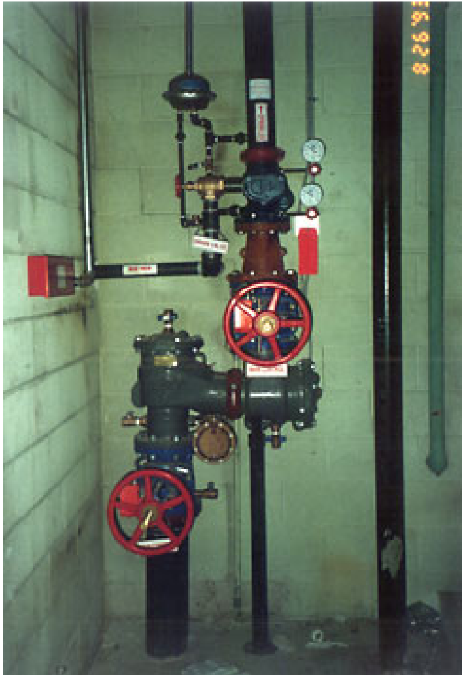
Example of an inline and vertical Reduced Pressure Backflow Assembly.
