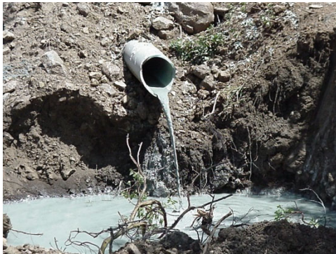
First Pit (heavy with cuttings)
