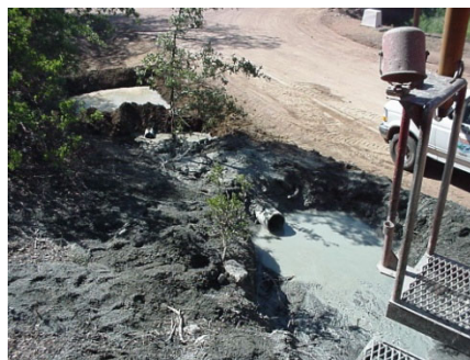
Constructed Mud Pits
