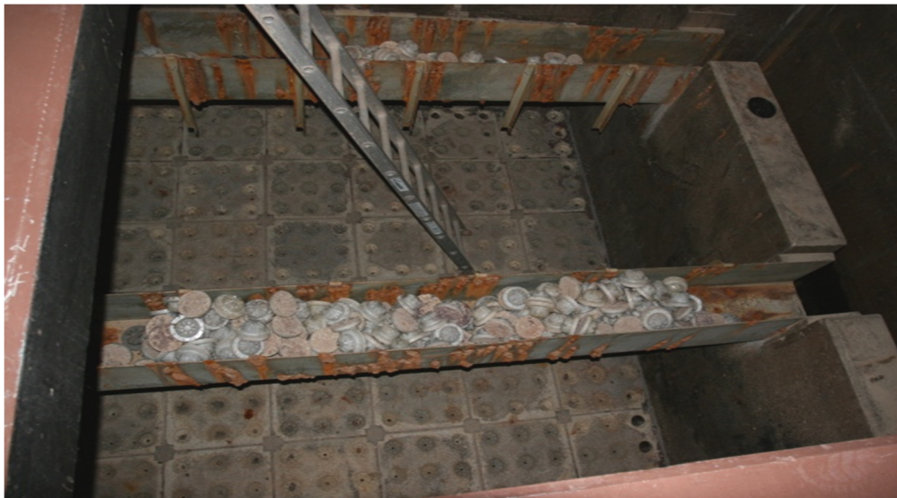
The photograph above shows a filter support bed under construction.
