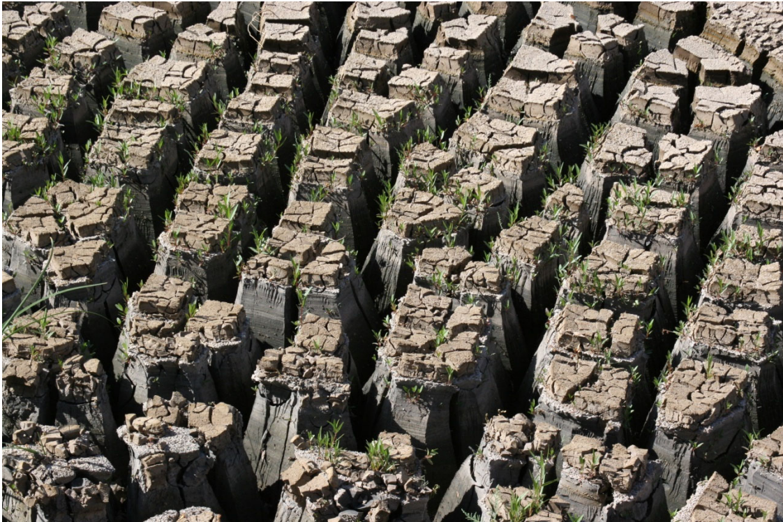
Pretreatment sedimentation basin, bottom photograph, sludge drying bed with new grass. Time to remove and dispose of this deep, dried sludge.
