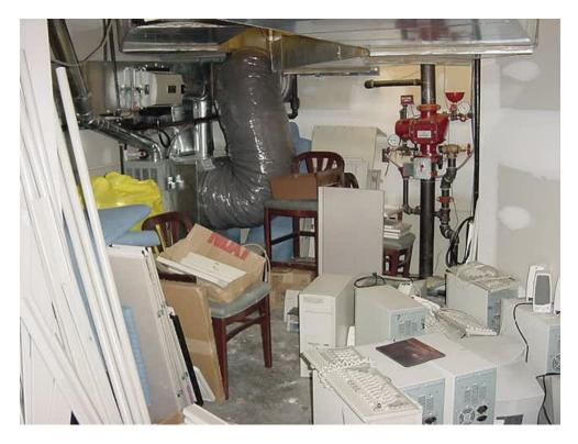
Notice the blocked access to the Fire Line Stand Pipe (Riser) and poor housekeeping. Depending upon the Fire Code, the Riser needs to be inspected at least annually or more frequently depending on the stock or processes in the facility. You will find a yellow inspection tag allow will spare sprinkler parts alongside or attached to the Riser.
