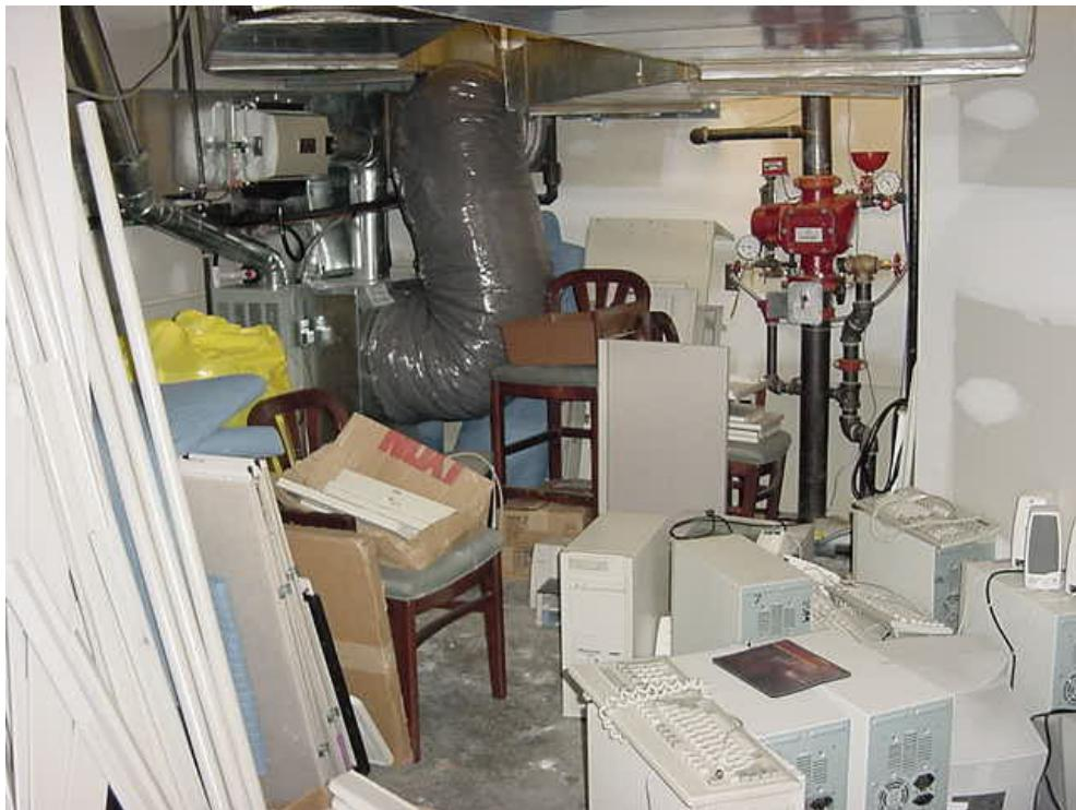
Notice the blocked access to the Fire Line Stand Pipe (Riser) and poor housekeeping. Depending upon the Fire Code, the Riser needs to be inspected at least annually or more frequently depending on the stock or processes in the facility. You will find a yellow inspection tag allow will spare sprinkler parts alongside or attached to the Riser.
