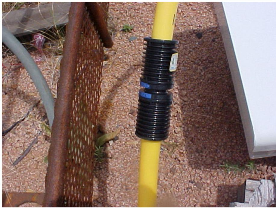
Mechanical (compression) joint on plastic gas pipe.
