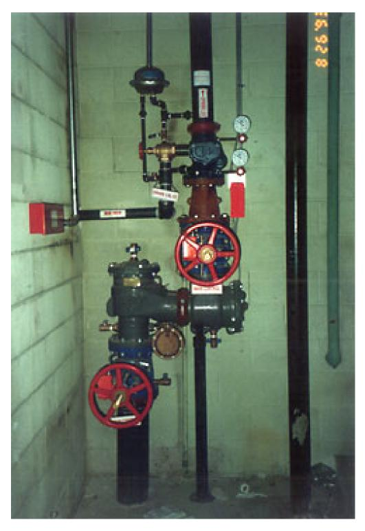
Reduced Pressure Backflow Assembly. A device to prevent contaminants from back flowing into the public water system.
