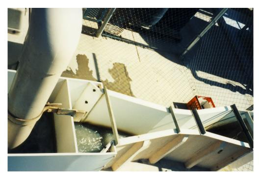
Compliance sampling flume used by commercial facilities for both water quality and volume.
