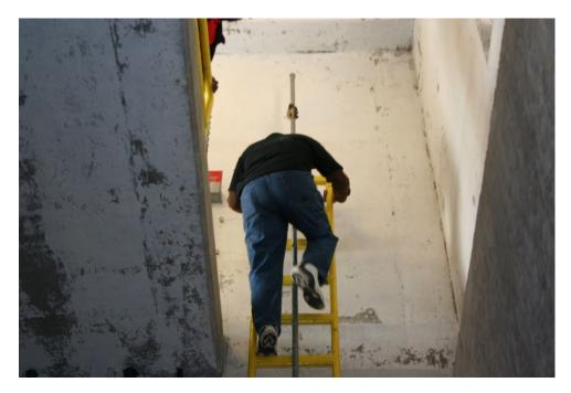
Never climb down a fixed ladder without a safety harness as this man is doing. Notice the steel support pole in the middle of the ladder.
