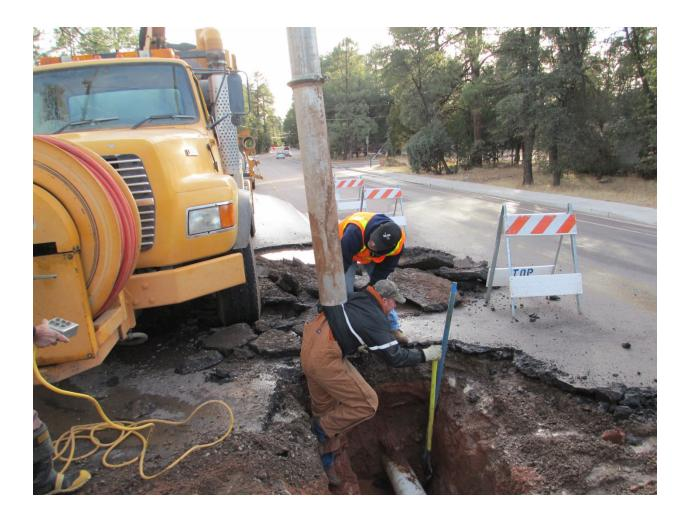
A vactor truck is often utilized in the pumping and cleaning of clogged sewer lines. Always be careful of all construction and maintenance concerns for everything in the sewer or septic field is dangerous and many operators have been injured and killed.
