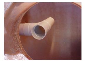
New fiberglass three compartment grease interceptor. You will need to fill the interceptor with water before connecting it to the sewer main.
