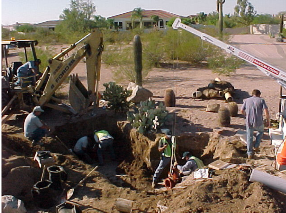
Top photo, two gate valves blew out, you can see the kickers or thrust blocks in the background.
