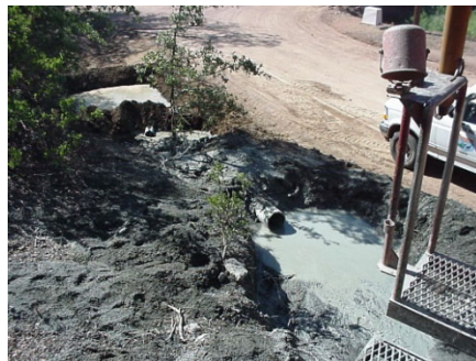
Constructed Mud Pits
