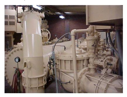
Looking inside of a booster pump station, notice the PRV and air relief valve.
