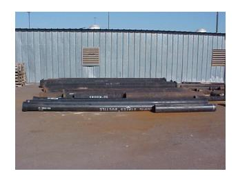
Ductile pipe cement-lined iron pipe shown above. I've seen thousands of dollars of pipe that is dropped or moved with the front bucket of a backhoe and destroyed. This destroys the interior protection of the pipe, causing leaks which will start in a few years. I know that some of you welcome this as job security.
