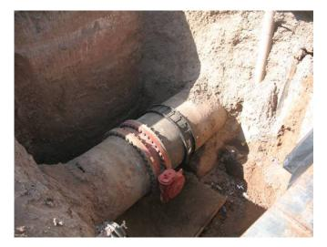
54 inch Butterfly valve on a huge transmission line. Nice job but no shoring, ladder or valve blocking.
