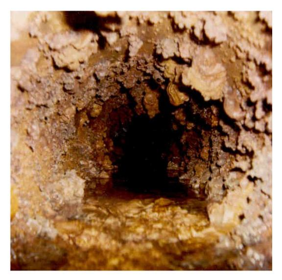
Notice the corrosion inside this cast iron main.
