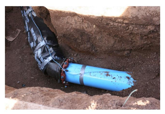
Photo of proper PVC to Ductile pipe with tracer wire and plastic installation. Notice restraing flang and missing poured kicker.
