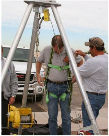
Donning the personal protective equipment (**PPE**) necessary for confined space entry.
