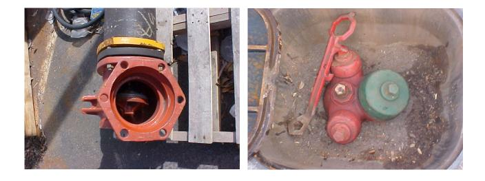
Left photograph-- the bottom of a dry barrel fire hydrant, there is a drainage hole on the back of this hydrant, sometimes referred to as a "weep hole". Right photograph-an "Airport Runway" type of hydrant.
