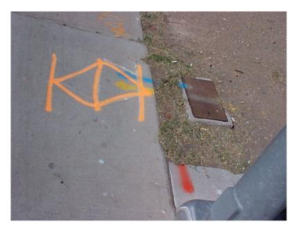
Red means-Electricity, Yellow-Gas, Blue-Water. It would be very difficult to replace this water service line because of all the buried utilities.
