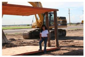
Shielding design and construction is not covered in the OSHA Standards. Shields must be certified in design by a registered professional engineer and must have
