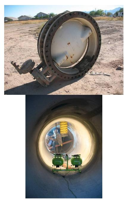
A broken 54-inch Butterfly valve and a worker inside the water main preparing the interior surface. Notice, this is a Permit Required Confined Space. A Hot work permit is also required.
