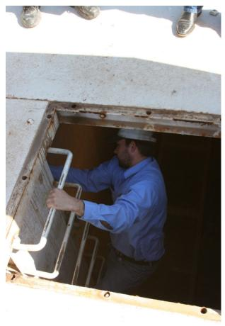
This situation appears as tanks within pits, pipe assemblies or vessels within pits, etc. In this situation, not only do the potential hazards associated with the outer confined space require testing, monitoring, and control, but those of the inner space also require similar procedures.
