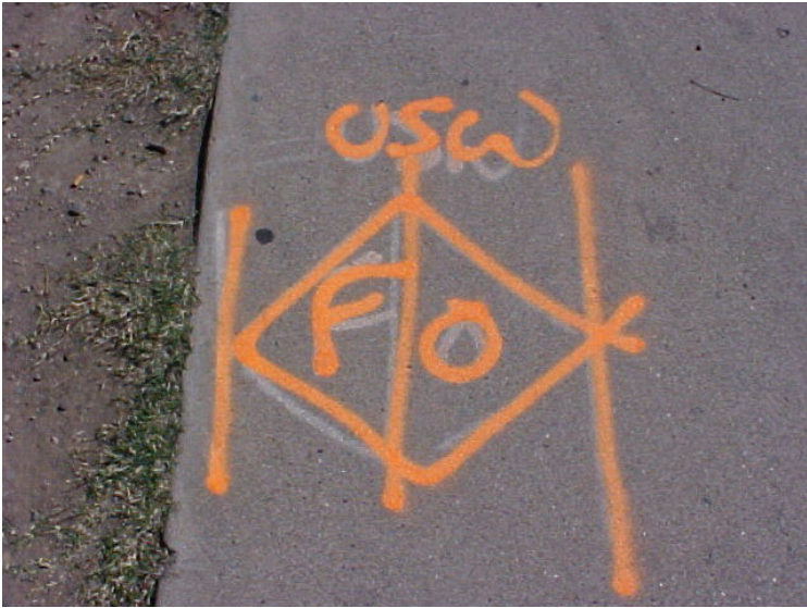
Orange spray marks represents - Telephone & Fiber Optics
