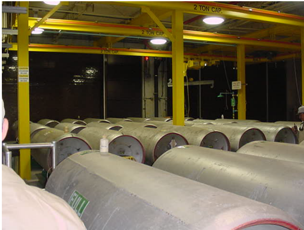
1-ton chlorine gas containers
