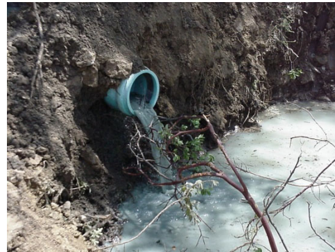
Last Pit (small amount of fines)
