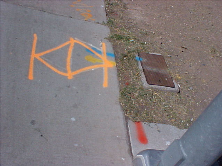
Red spray marks represents - Electricity, Yellow represents-Gas, Blue represents-Water
