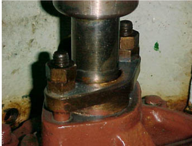
PUMP PACKING BOX WITH ADJUSTMENT LOCK NUTS
