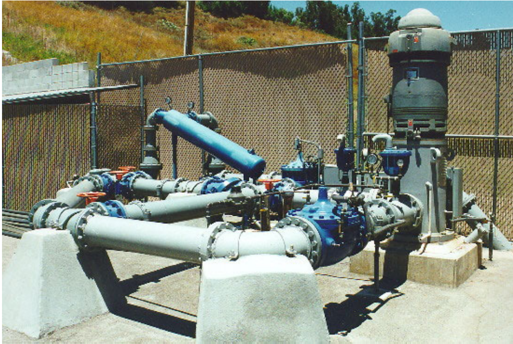
VERTICAL TURBINE WELL EXAMPLE
