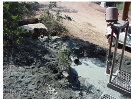
Constructed Mud Pits
