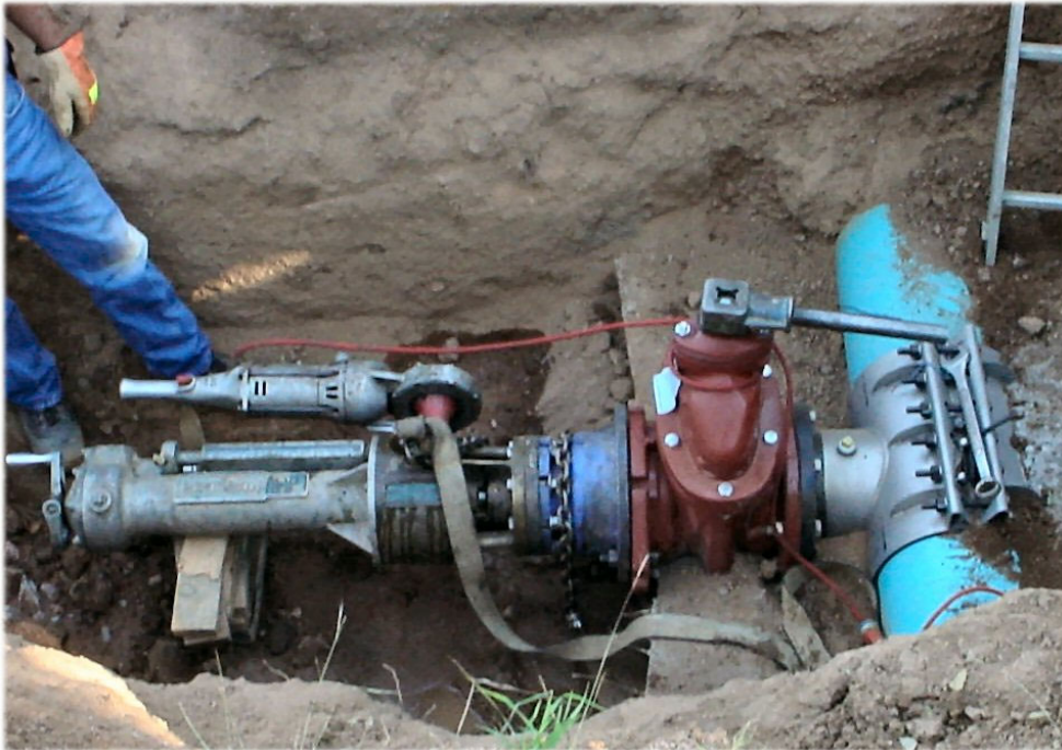
Bottom photo, a tapping machine and a new gate valve. These tapping machines are very expensive.
