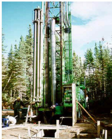
Wire wrapped screen being installed in a well.
