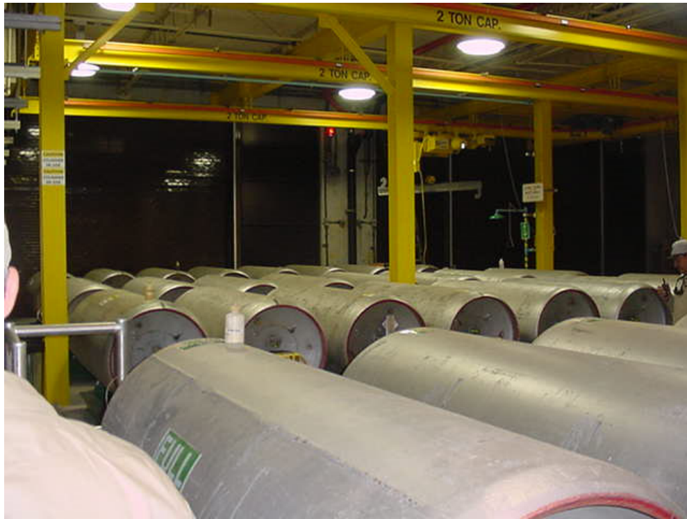
1-ton chlorine gas containers
