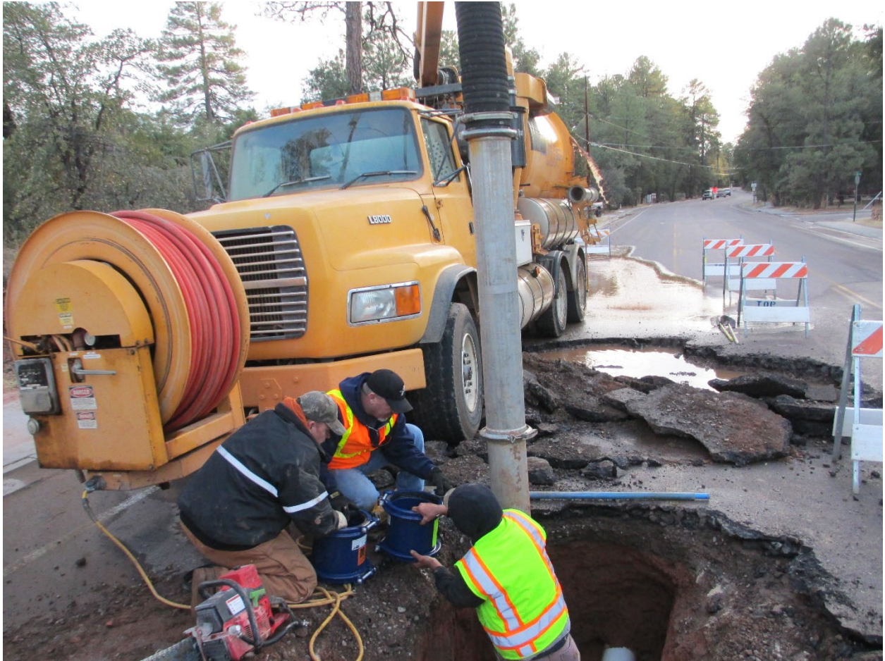
A normal day of work for most distribution system operators. Using a Vector to pump out the hole while replacing a plastic main section.
