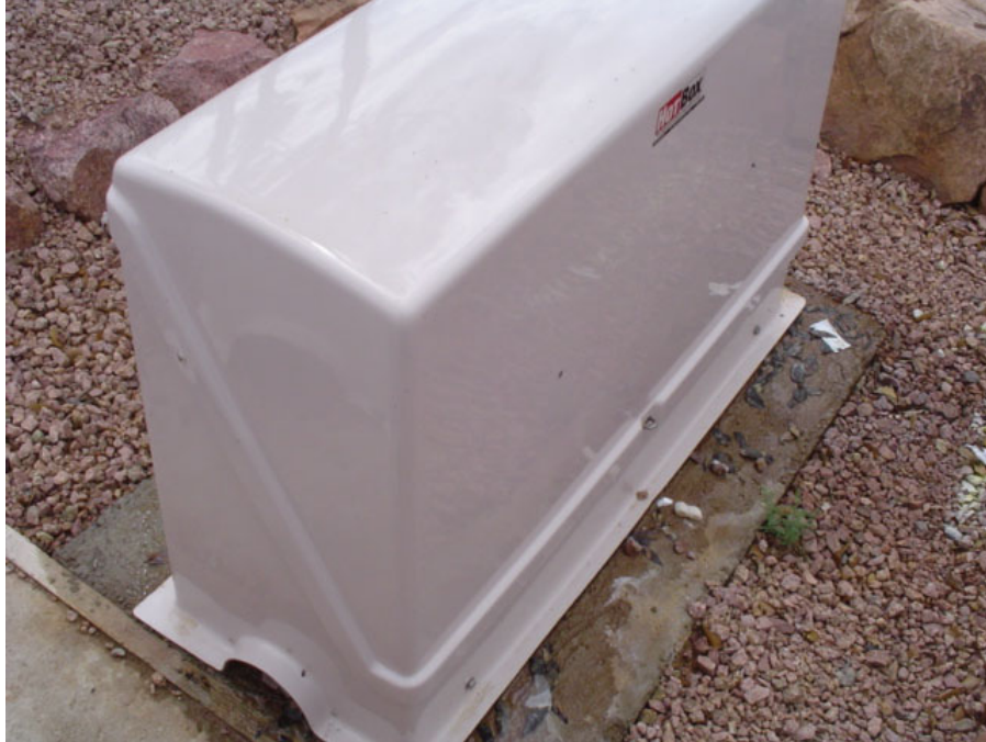
Top photo, a Hot Box, a good method of keeping the assembly from freezing during the winter. Bottom, electrical heat tape method for freeze protection.
