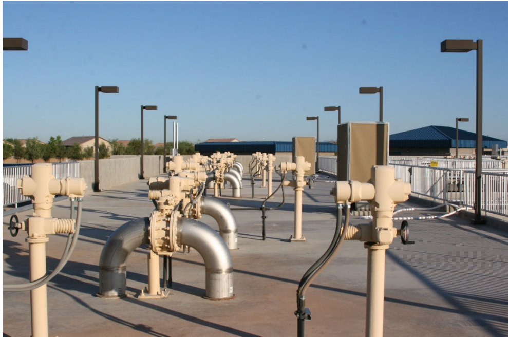
At a water treatment plant, we can see both valve actuators control devices and Butterfly valves as well. Bottom photo is a cut-away of an actuator.
