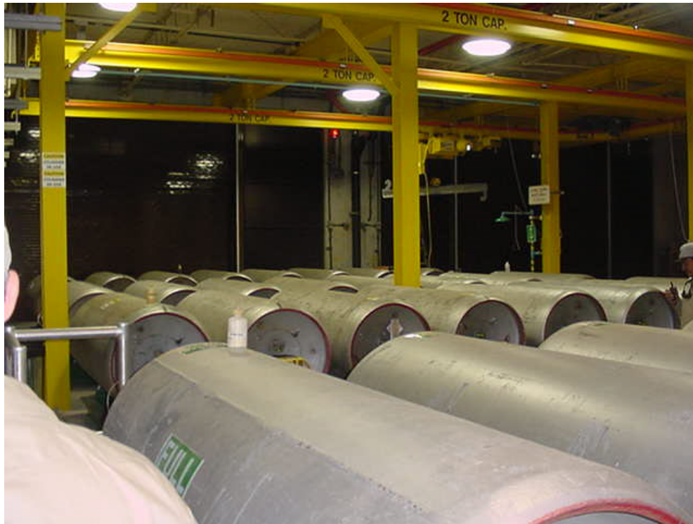
1-ton chlorine gas containers
