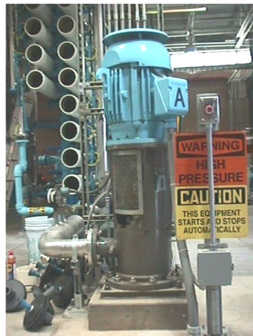
Membrane Filtration System
