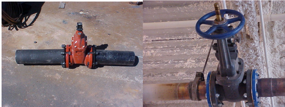
Different types of Gate Valves. (Linear)
