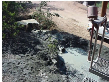
Constructed Mud Pits
