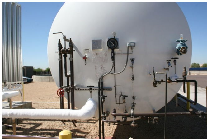
Oxygen tank is necessary to generate O 3
