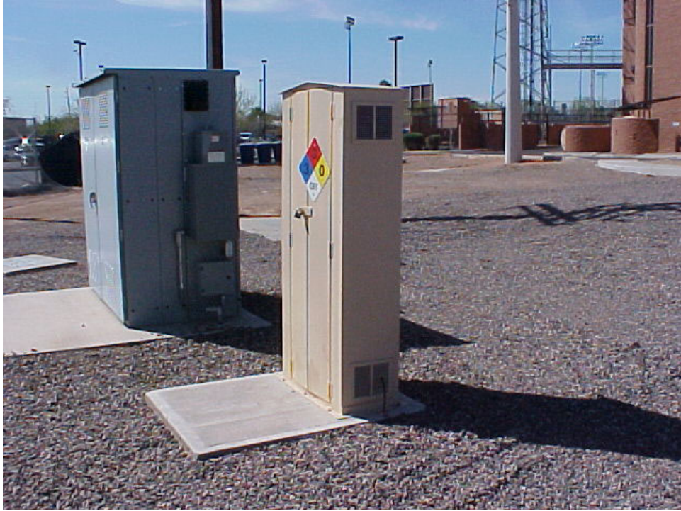
Small chlorine storage shed in the foreground; notice the vents at the bottom and top. The bottom vent will allow the gas to ventilate because \text{Cl}_2 gas is heavier than air.
