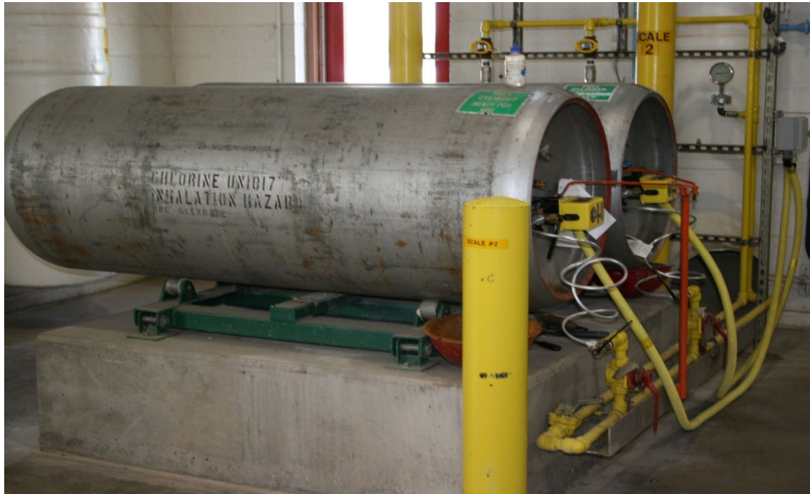
1-ton chlorine containers. Automatic shutoff device connected to the liquid side only. The top valve is used for the gas. Remember that containers lay on their sides and cylinders stand upright. Roller bearings should not be used to rotate the container because of the ease of rotation is too great.
