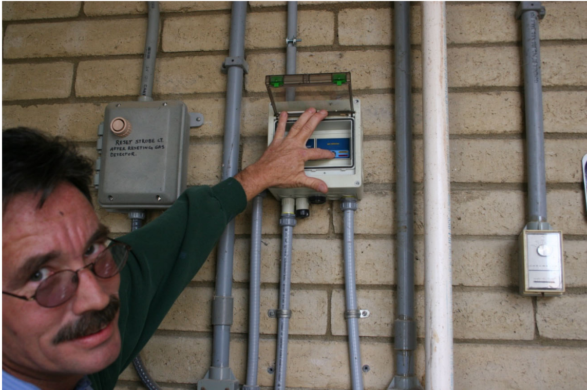
Top photograph, adjusting the chlorine leak alarm sensor. Bottom photograph, chlorine container weight scales.
