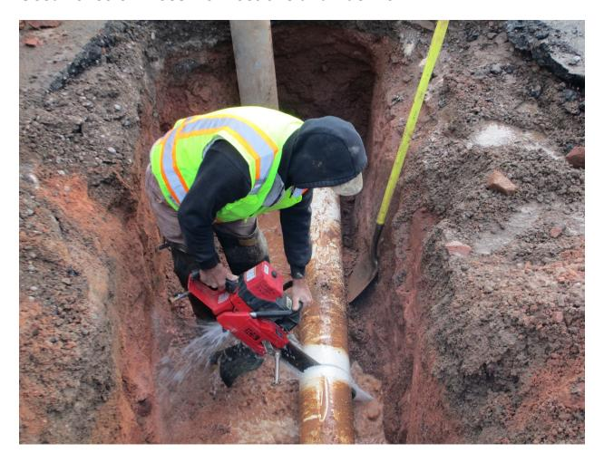
Cutting out a damaged water main section.
