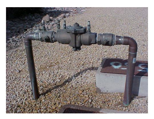
**Leaky RP**--have your assemblies tested annually or more often. Re-test after repairs and problems. A RP should not leak more than 1 or 2 minute—any more than that, there is a problem; a piece of debris or stuck check is causing the RP's hydraulic relief port to dump.
