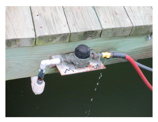
The above photo is of a unprotected water meter at a boat dock.
