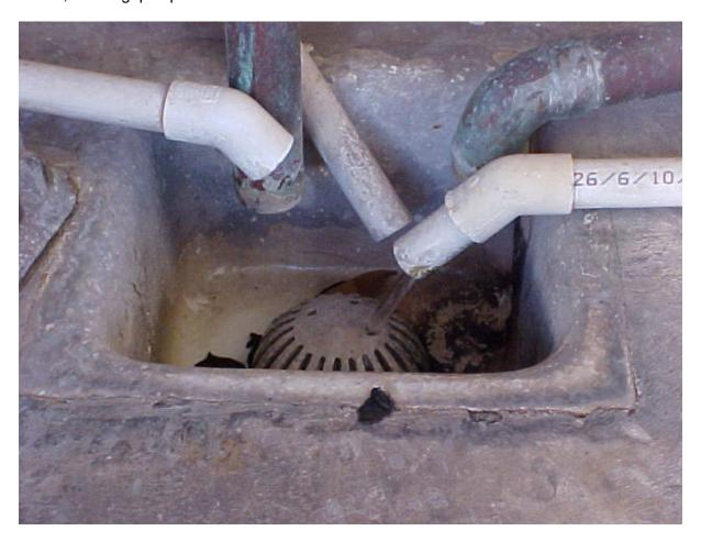
Which of these ice machine drains has an approved air gap? Here is a better question; would you use the ice from this ice machine? This is where all those stories about cockroaches and stomach flu originate.
