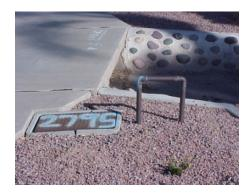
I've seen this type of poor installation many times and is a common site because of uneducated Inspectors and/or backflow personnel. This line feeds an irrigation system, no protection at all and was in place for many years.
