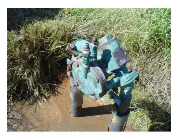
Here is an RP that had never been tested and leaked every day until the grass was 3 feet high and the owner notified the Water Department of a water leak. The water meter reader should have caught this problem in the first couple months.
