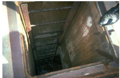
This space requires an emergency retrieval system, continuous air monitoring, and safety watch or two-way communication for safe entry.
