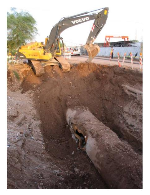
54-inch water main blow out. Are you prepared to handle this type of an emergency? Most water providers will have to contract this type of work out because they are not prepared.
