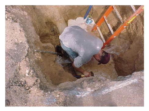
We have a ladder, but no protective system in place or hardhat. Is that Asbestos? Sure looks like it and it is not taped up as OSHA requires.
