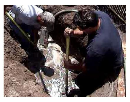
Remove employees from the trench when there are indications of possible caveins, protective system failures, or other potentially hazardous conditions. Never work in water without proper protection. You will have to wear a Lifeline with a rope to drag your dead body out of these hazardous conditions.
