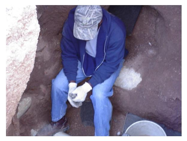
This poor soul is probably going to be a short timer here on earth. He is sitting on the sewer main in a bell shaped hole under a steel plate which cars are driving over. No protection at all. There was a ladder in the trench was about 50 feet away. He wouldn't make it out of a cave-in unless he had wings.
