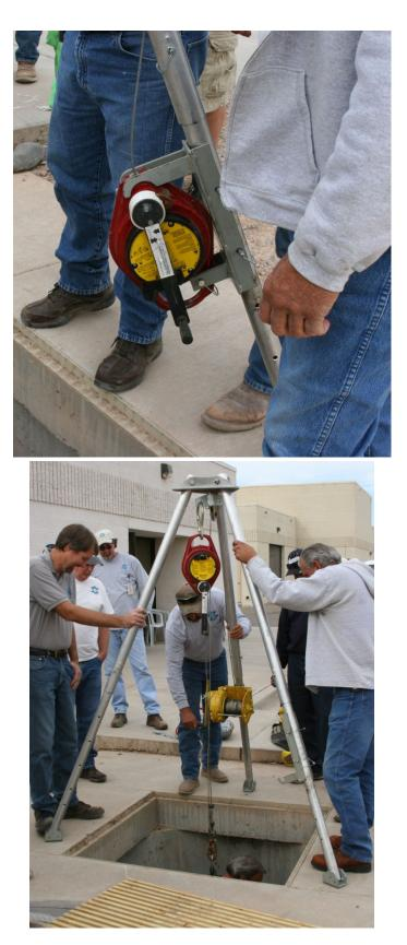
Checking the cable tension and inertial locking mechanism of the retrieval assembly.
