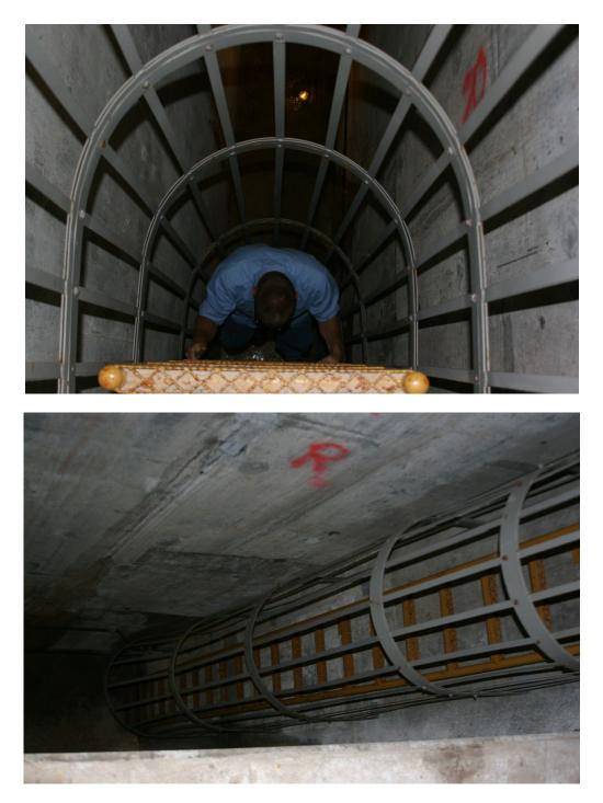
**Scenario.** A fixed ladder drops deep inside a permit required or type II confined space. One man goes inside and passes out from hazardous fumes. A second man goes in and dies within seconds trying to help his buddy.
