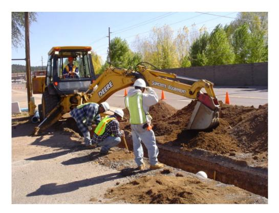
Two unsafe excavation examples: Top, notice the man in a 6-foot-deep trench with no ladder or shoring, and the placement of spoil. Bottom picture, utilities are marked after the excavation has begun, no hard hats, no ladders, no protective system, incorrect spoil placement.
