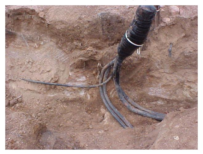
Telephone Cables, difficult to dig around, just as with as electrical lines.
