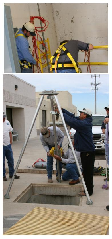
Example of a "*D-Ring*" and fall protection harness used when entering a confined space. The D-Ring provides a compatible anchor point for connecting devices such as lanyards or retractable lifelines. The shock absorbing lanyard provides a deceleration distance during a fall to reduce fall arrest forces for extra protection against injury.
