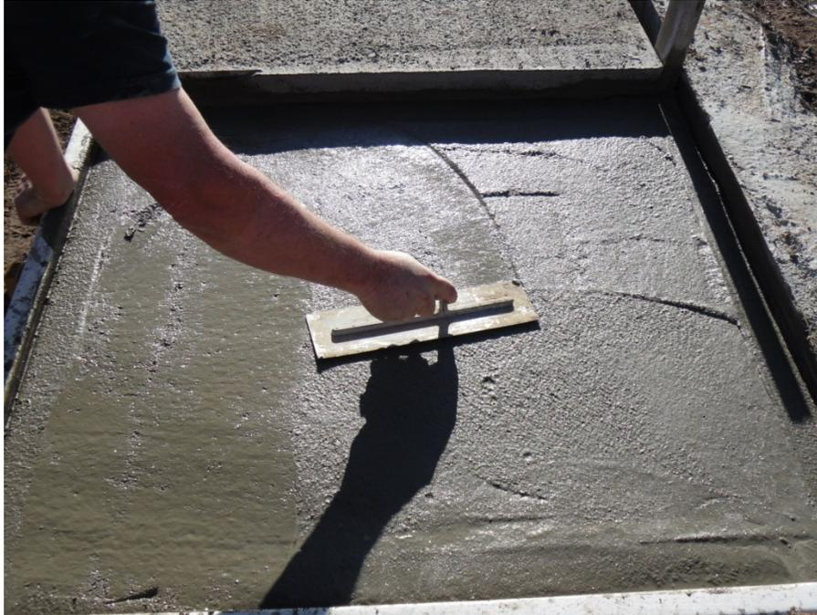
Using a hand float to smooth out the cement. I suggest allowing the pour to set up in about one hour and start the final finish. This period is dependent on the weather and you can generally tell how the mud is setting up by the amount of water or fat on the top. I like to wait until the excess water is gone but the white or dry cement is not beginning.
