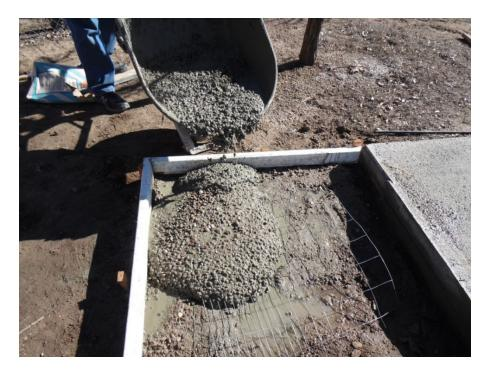
Top: Pouring the mud in  $2 \times 4$  form. It is good to place steel hog wire or re-bar to reinforce the pour and keep the pad from cracking. Bottom: Using a  $2 \times 4$  to level and tamp the cement. You can actually finish the cement with a board and give a broom finish to top. I suggest an edger tool or you'll have sharp edges. A sharp edge is okay in a farm setting to help wipe of boots.
