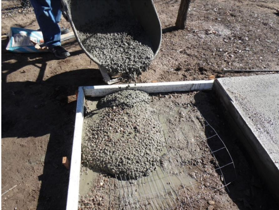
Top: Pouring the mud in 2 x 4 form. It is good to place steel hog wire or re-bar to reinforce the pour and keep the pad from cracking. Bottom: Using a 2 x 4 to level and tamp the cement. You can actually finish the cement with a board and give a broom finish to top. I suggest an edger tool or you'll have sharp edges. A sharp edge is okay in a farm setting to help wipe of boots.
