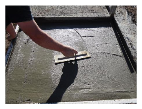
Using a hand float to smooth out the cement. I suggest allowing the pour to set up in about one hour and start the final finish. This period is dependent on the weather and you can generally tell how the mud is setting up by the amount of water or fat on the top. I like to wait until the excess water is gone but the white or dry cement is not beginning.
