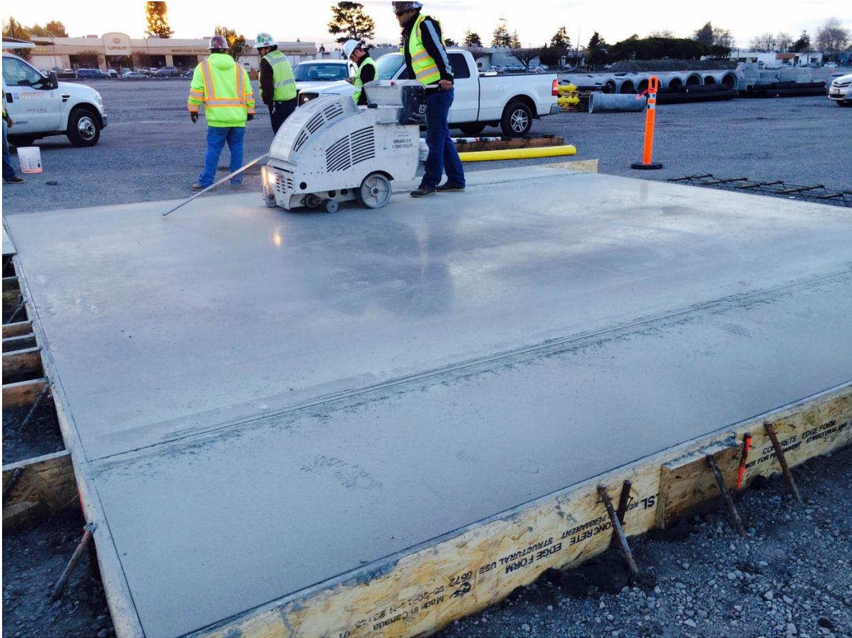
**Saw cutting expansion joints in a fresh pour.**
