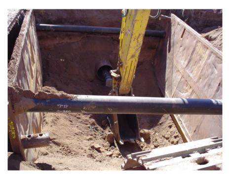
**OSHA Violation--**No ladders, but the best part is the homemade trench box using waterlines as the cross-braces. Remember, trench boxes and shields are a manufactured and engineered safety device that cannot be modified, especially by the competent person. This box collapsed in the hole. Workers must enter and leave the shield in a protected manner, such as by ladder within the shield or a properly sloped ramp at the end.
