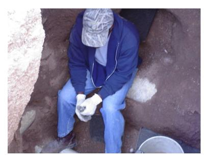
**OSHA Violation.** It is difficult to see, but this poor soul is inside a death trap. He is in a deep trench sitting in a bell-shaped hole, sitting on a sewer main. He has good shade from a steel plate that is covering the road with cars driving on top. No protection at all. There was a ladder about 50 feet away. Good luck!
