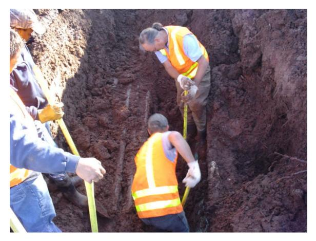
How would you make this excavation safe to work inside? The trench is 9 feet deep. OSHA Violations include no hard hats, no ladders, and no daily inspection form.
