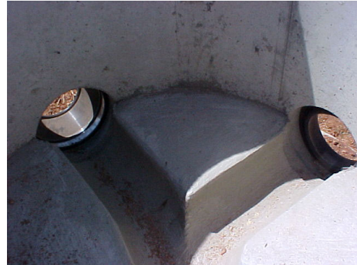
New sewer manhole with sewer mains before final burial.
