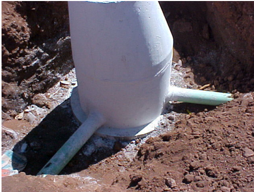
New sewer manhole with sewer mains before final burial.
