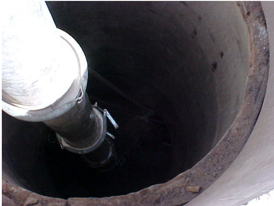
A Vactor clearing a Manhole.
