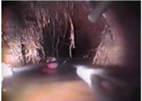
joint, tree roots will penetrate the opening to reach the nutrients and moisture inside the pipe. This phenomenon continues in winter even though trees appear to be dormant.
