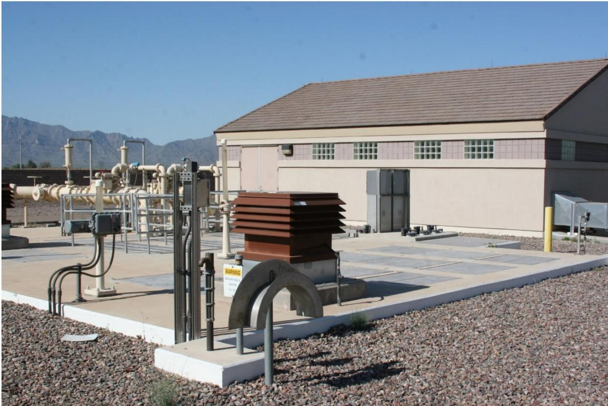
Wastewater lift stations are facilities designed to move wastewater from lower to higher elevation through pipes. Key elements of lift stations include a wastewater receiving well (wet-well), often equipped with a screen or grinding to remove coarse materials; pumps and piping with associated valves; motors; a power supply system; an equipment control and alarm system; and an odor control system and ventilation system.
