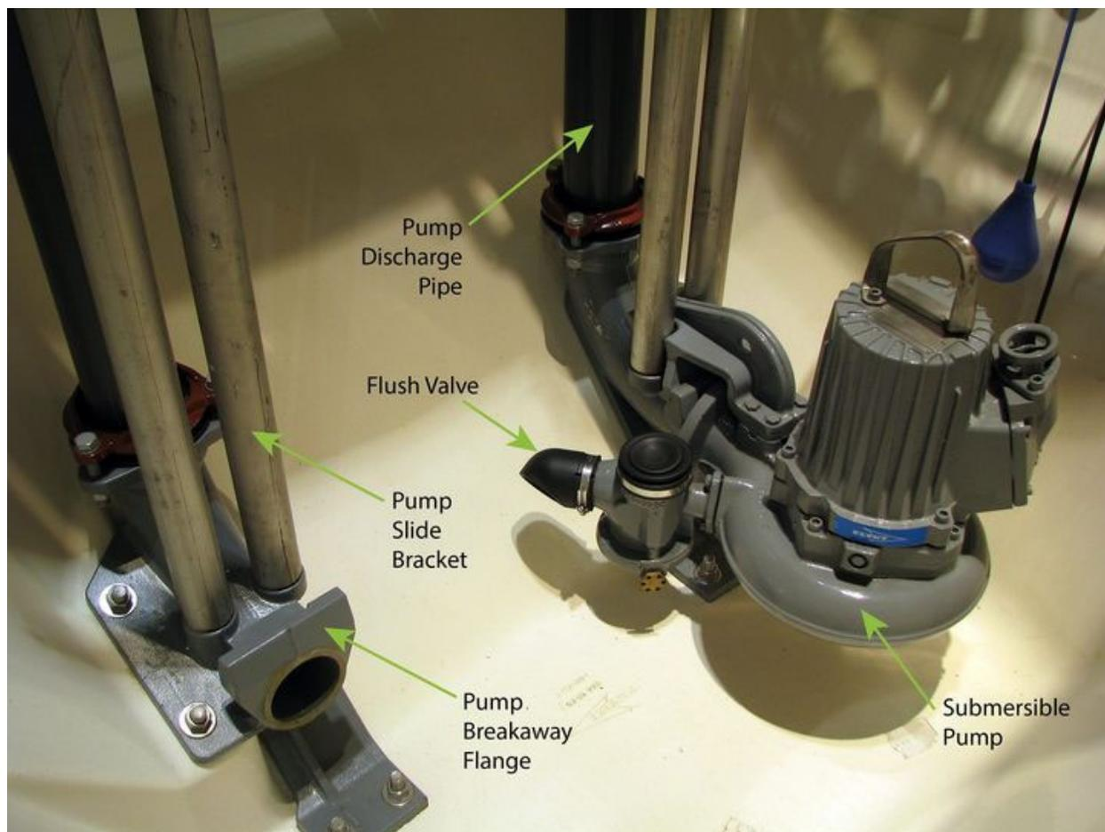
Depending on the system, the pumps are designed to run at a reduced rate. The pumps may also alternate to equalize wear and tear. Additional pumps may provide intermediate capacities better matched to typical daily flows. An alternative option is to provide flow flexibility with variable speed pumps.
