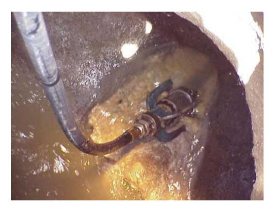
This is a sewer line that has a large amount of grease buildup that will be cut out. Grease gets into the sewer line by pouring grease left over from cooking, down the kitchen sink.
