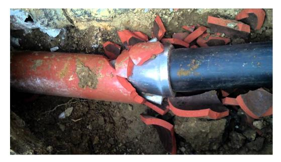
Old sewer lines are often made of cast iron and clay. These old sewer lines eventually crack and fail to drain properly. Roots and debris make their way into old sewer lines causing repeated obstructions and service calls.
