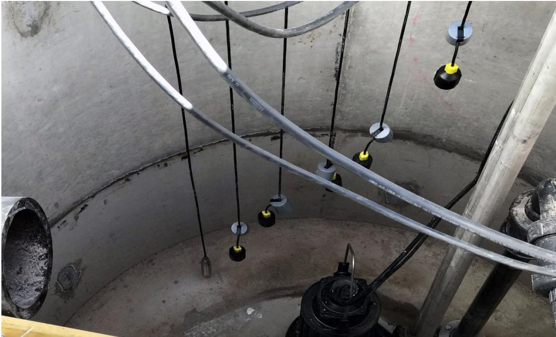
Other control alternatives include electrodes placed at cut-off levels, floats, mechanical clutches, and floating mercury switches.
