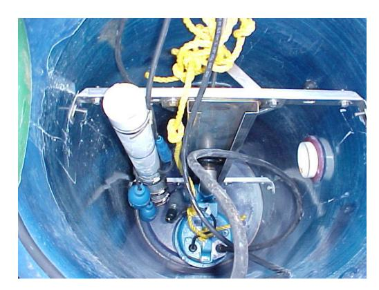
Low-Pressure System Inside a grinder pump found outside a home, the inlet is 3 inches and outlet is only  $1^{1}/_{2}$  inches.
