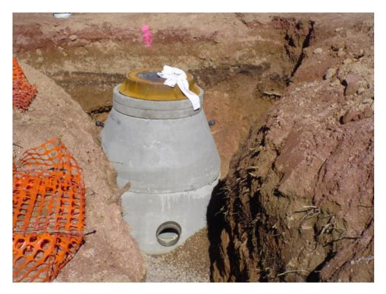
Top photograph, new manhole. Bottom, a repaired sewer main after being damaged by the water distribution department using a backhoe without locates.
