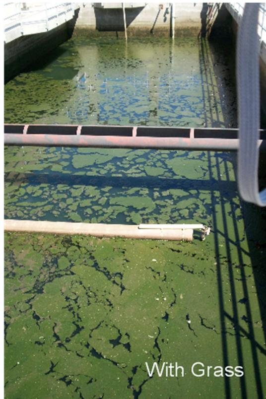
Sewer filled with grass will damage your system, pumps, and upset the wastewater treatment system. Require your industrial users like golf courses to install grass, grease, and sand/oil interceptors.
