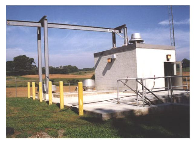
**Lift Station**: A facility in a sewer system consisting of a receiving chamber, pumping equipment, and associated drive and control devices which collect and lift wastewater to a higher elevation when the continuance of the sewer at reasonable slopes would involve excessive trench depths; or that collects and raises wastewater through the use of force mains from areas too low to drain into available sewers. There should not be an odor coming from a Lift Station.
