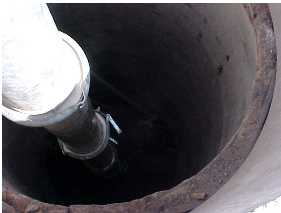
A Vactor clearing a Manhole.
