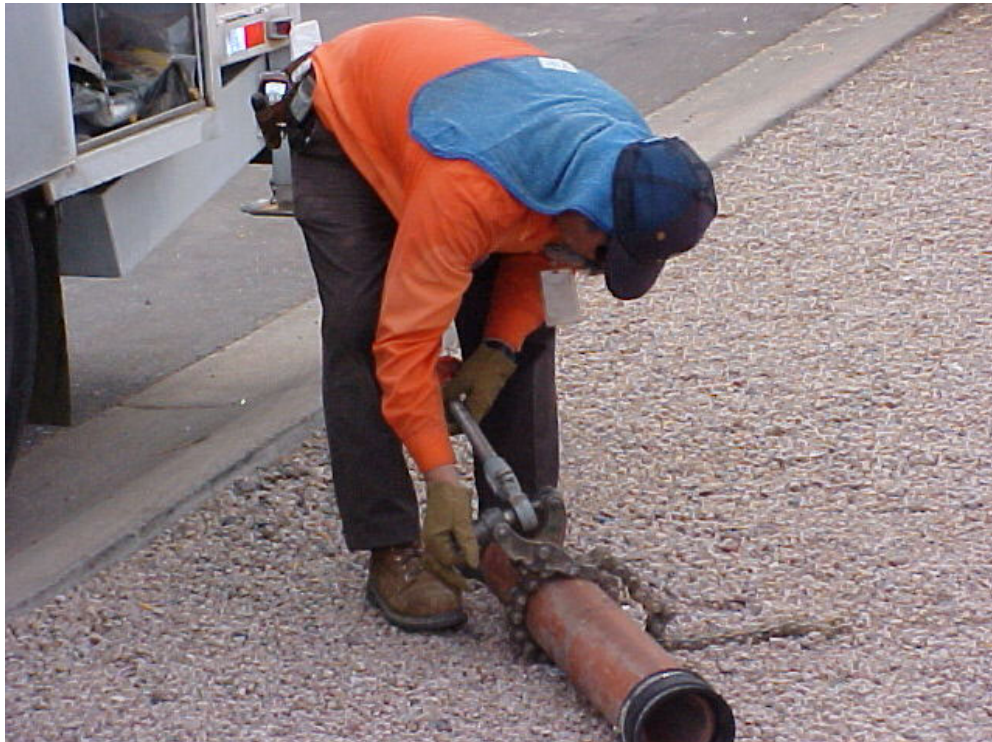
Using chain nubbars to cut pipe.
