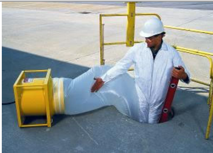
Forced air ventilation with a disposable air shaft.
