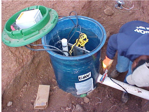
Installation of grinder pump for a low-pressure system.
