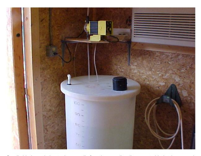
Small chlorine solution tank, normally found on small wells or post-chlorination areas in the disitribution system
