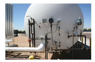
Oxygen tank is necessary to generate O<sub>3</sub>
