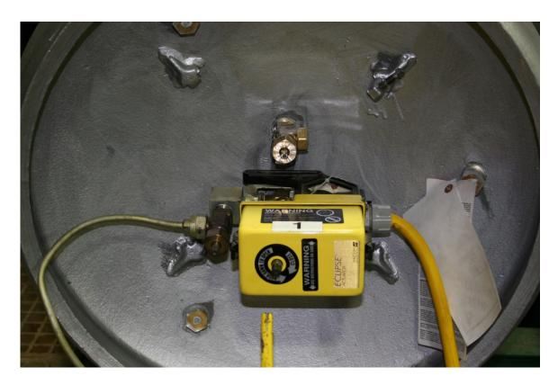
1-ton chlorine containers. Automatic shutoff device connected to the liquid side only. The top valve is used for the gas. Remember that containers lay on their sides and cylinders stand upright. Roller bearings should not be used to rotate the container because of the ease of rotation is too great.
