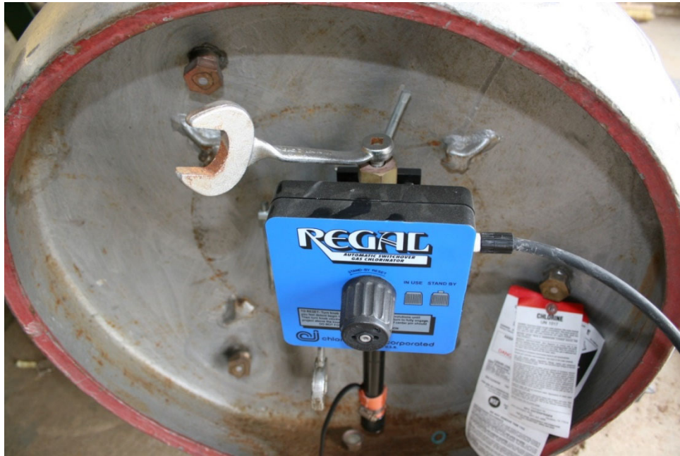
Top photograph, this blue device prevents the liquid from being pulled and freezing the lines. Bottom photograph, the application of an ammonia mist to detect a chlorine gas leak. Notice that employee is not wearing required PPE.
