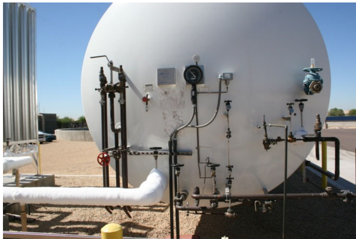
Oxygen tank is necessary to generate O 3
