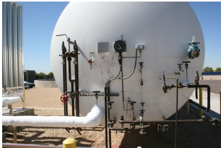
Oxygen tank is necessary to generate O 3
