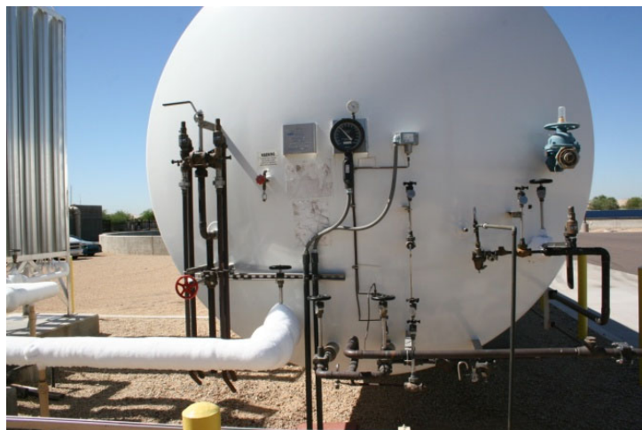
Oxygen tank is necessary to generate O 3
