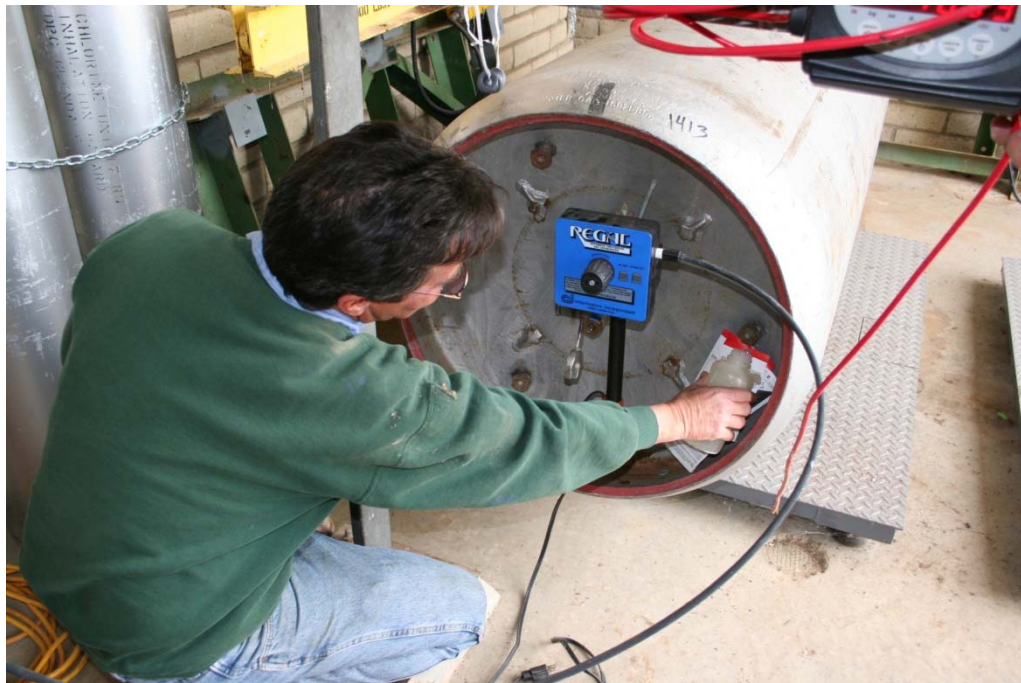
Top photograph, this blue device prevents the liquid from being pulled and freezing the lines. Bottom photograph, the application of an ammonia mist to detect a chlorine gas leak. Employee is not wearing any required PPE.
