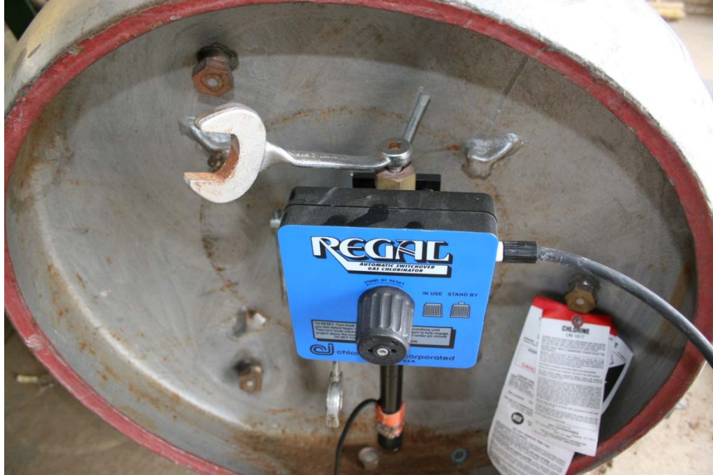
Top photograph, this blue device prevents the liquid from being pulled and freezing the lines. Bottom photograph, the application of an ammonia mist to detect a chlorine gas leak. Employee is not wearing any required PPE.
