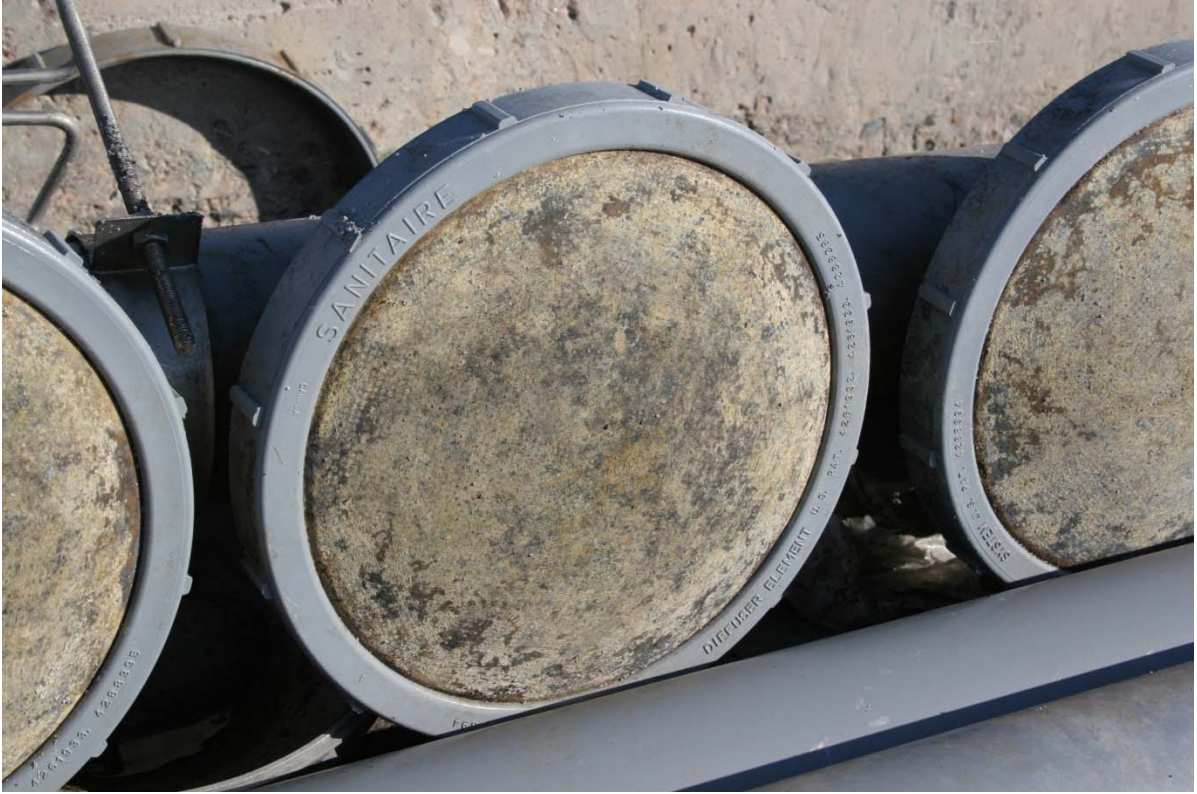
Here is a rare and up-close view of non-porous diffuser heads. Notice the heads that are missing in the bottom photograph.
