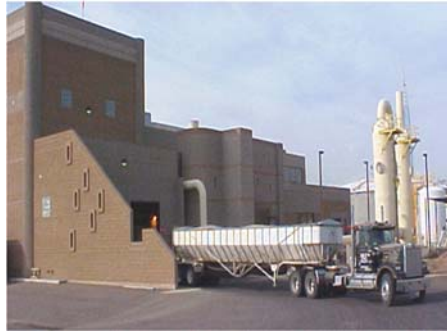
Large solids treatment facility
