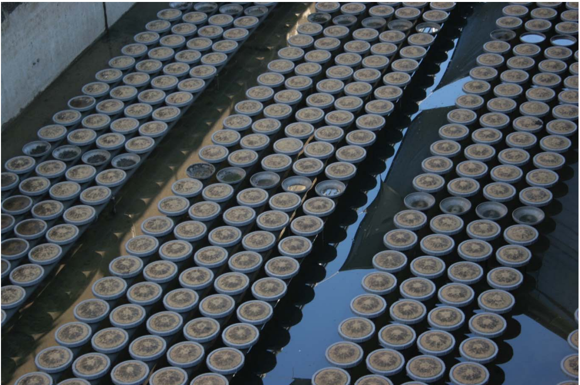
Here is a rare and up-close view of non-porous diffuser heads. Notice the heads that are missing in the bottom photograph.
