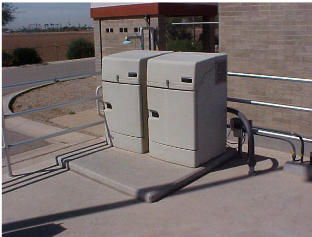
Two automatic wastewater samplers, one for Local Limits or compliance and the other for the wastewater plant operator to determine plant efficiency.
