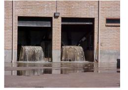
Domestic waste overflow at a WWTP headworks. Sometimes headworks do overflow, usually due to rags, grease and debris, or operator error. We do not like to see this happening!
