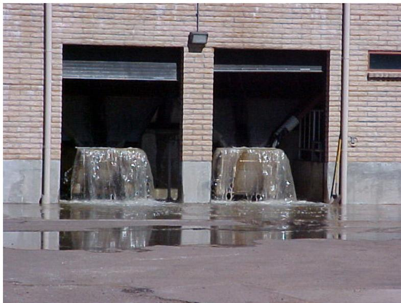
Headworks flooding or overflowing because of high grease (FOG) loading.
