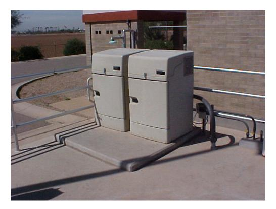
Two automatic wastewater samplers, one for Local Limits or compliance and the other for the wastewater plant operator to determine plant efficiency.
