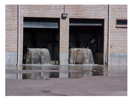
Headworks flooding or overflowing because of high grease (FOG) loading.
