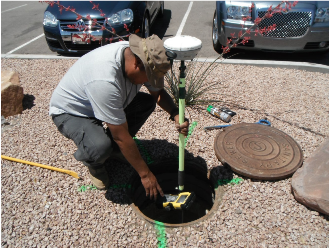
Marking the GIS of the sewer main for proper mapping and identification purposes.
