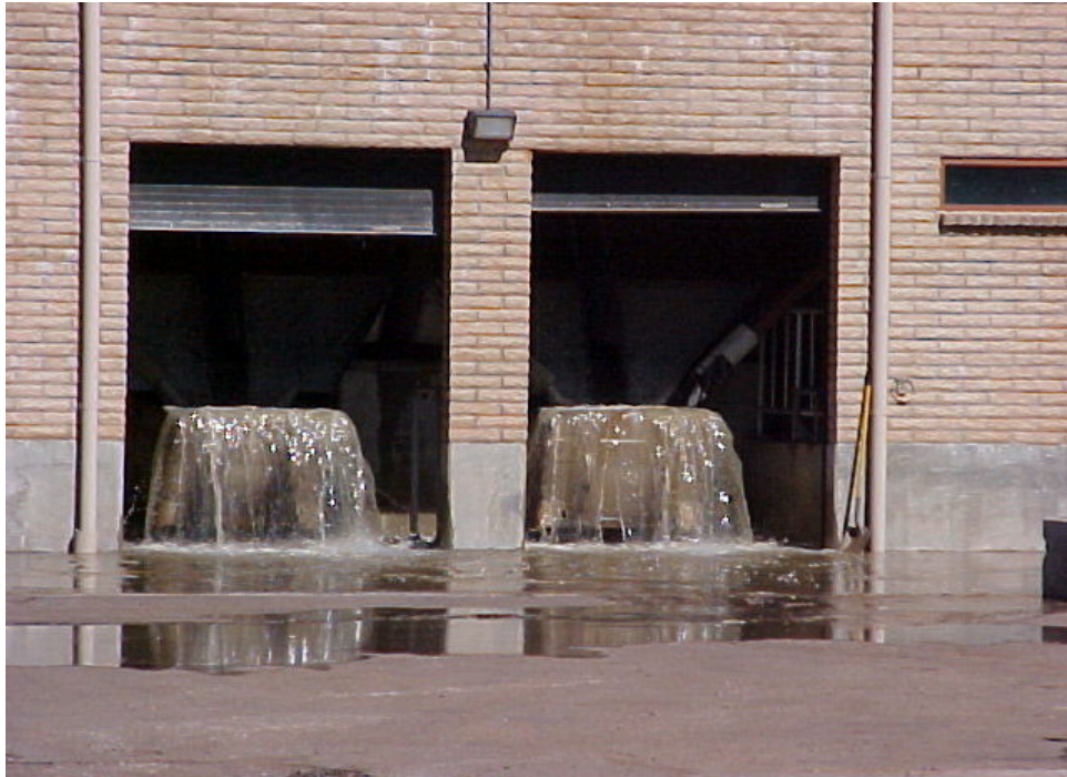
Effects of a clogged bar screen causing Headworks to flood. This mess was caused by grease clogging and happens frequently.
