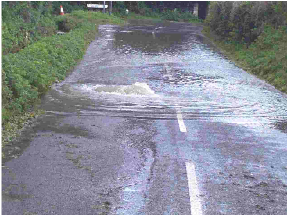
Sewer Manhole surcharged due to grease plugging the sewer line. Both of these problems can result in the Operator being fined and/or charged with a criminal offense. Most States will fine the Operator and/or not the City or Company.
