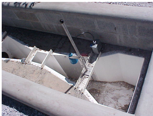
Parshall Flume and Ultrasonic Flow Meter Notice the debris and most POTW's will write a NOV for uncleanness.
