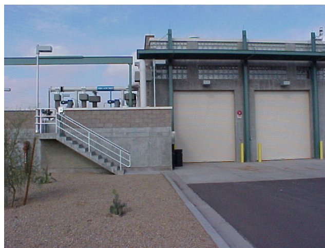
Wastewater Treatment Headworks
