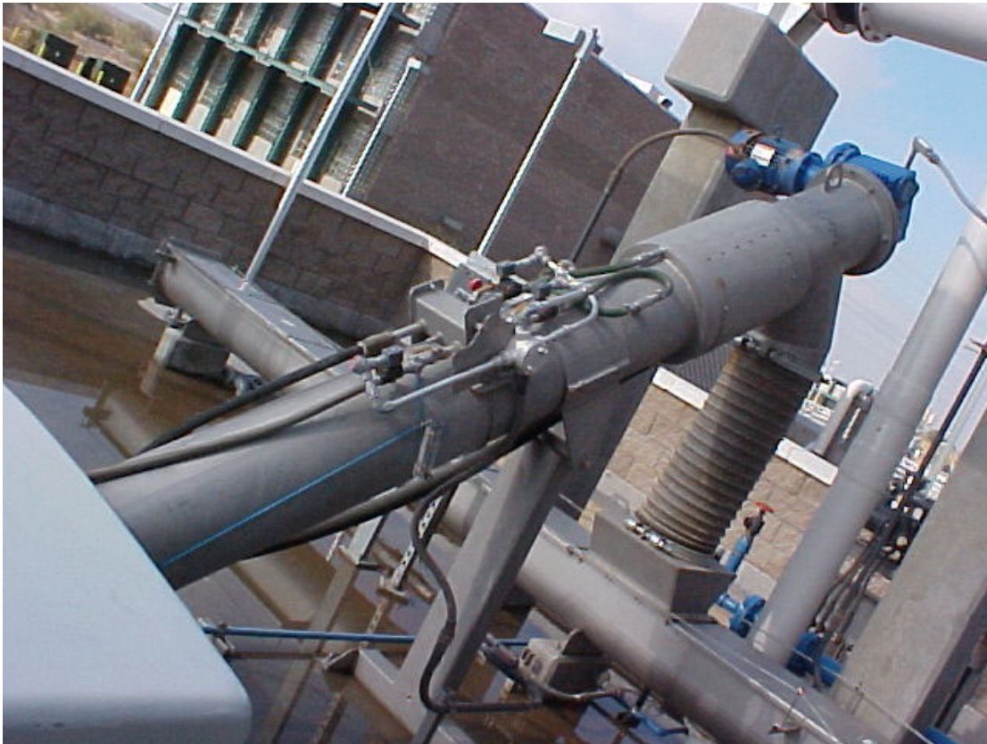
Rotating Bar Screens The Wastewater Headworks is a key compliance sampling location.
