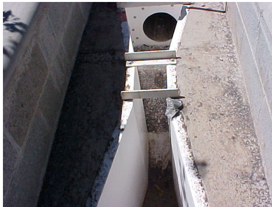
Parshall Flume and Ultrasonic Flow Meter Notice the debris and most POTW's will write a NOV for uncleanness.
