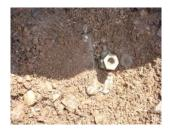
Another buried RP assembly deep inside a vault, all we can see is a test cock. All RPs need to be installed 12 inched above the ground. This device was buried in ground and not tested for over 25 years. Owners are required to test their devices once a year at a minimum.
