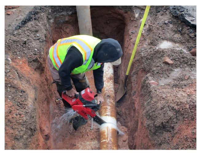
Cutting out a damaged water main section.
