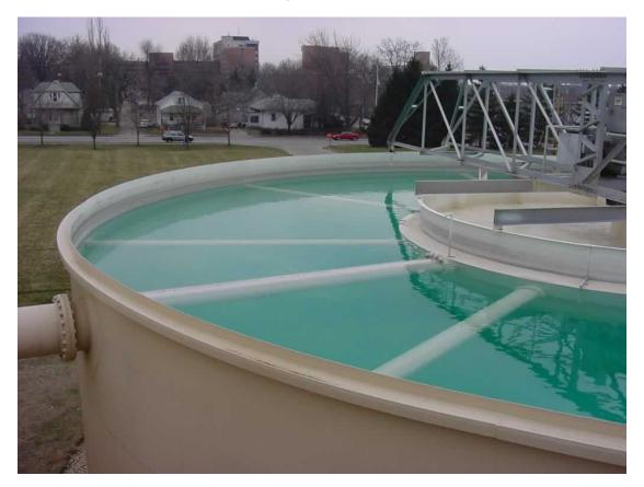
One of the steps in water treatment is softening. Lime can be added to the water, resulting in an exothermic reaction and a pH increase to 11.
