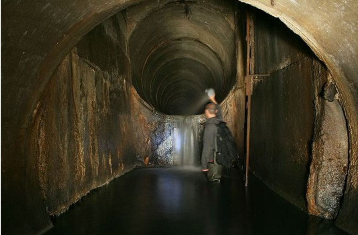
Inside a large sewer main looking for cockroaches.
