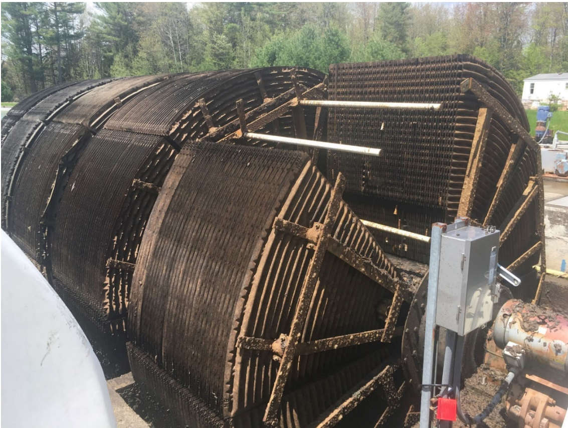
An RBC with one section removed.
