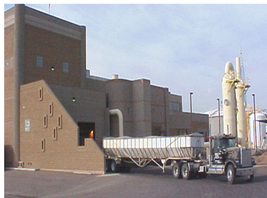
Large solids handling facility
